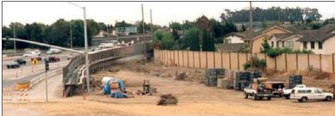
Existing noise barrier left in place until replacement noise barrier is constructed
